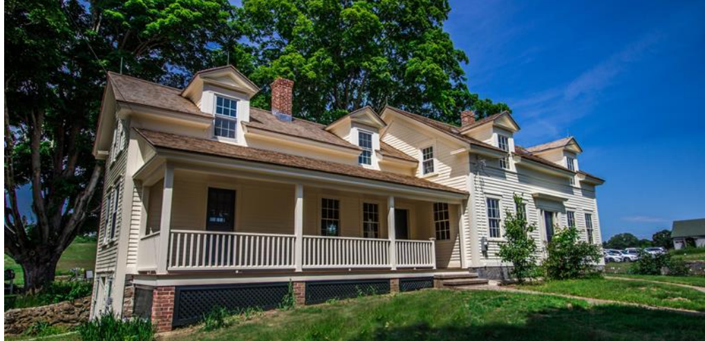
Farmhouse at Franklin Farm (ca. 1857, Cumberland), before and after State Preservation Grant-funded exterior restoration.
