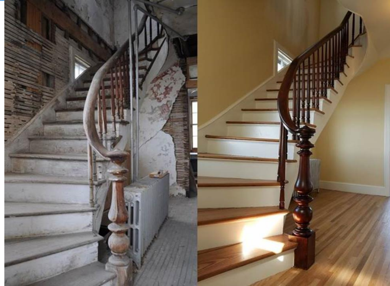
Pomham Rocks Lighthouse (1871, East Providence), before and after State Preservation Grant-funded interior restoration.
