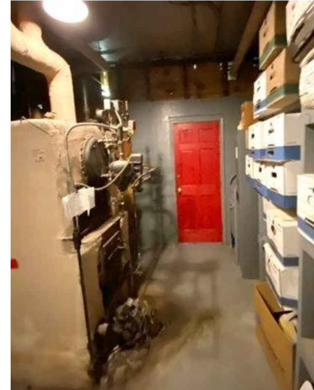
Hope Valley Barracks Boiler, Evidence Room & File Storage
