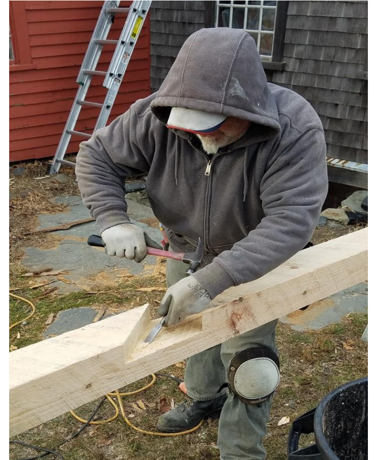
A craftsman hand-notches a rafter for the State Preservation Grant-funded roof restoration at the Coggeshall Farm Museum (c. 1799, Bristol).
